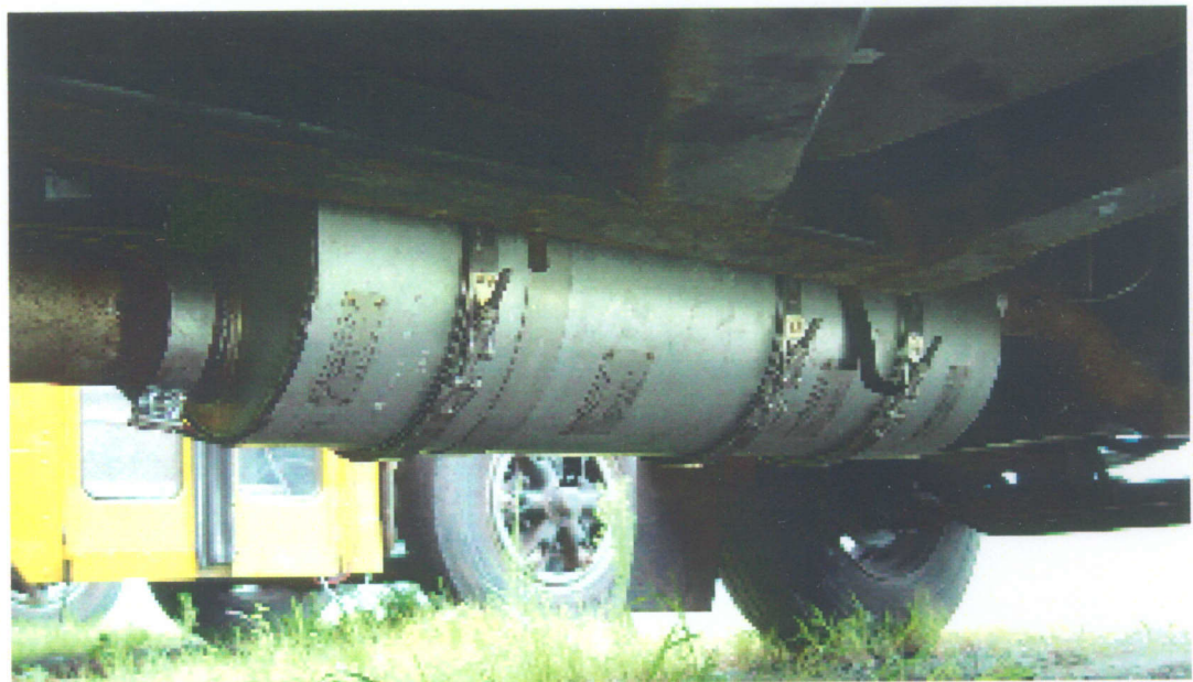
Figure 9: JMI CRT installed into the exhaust system of a DT466E school bus engine prior to mobile testing.
